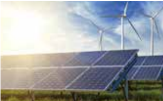
New energy photovoltaic
